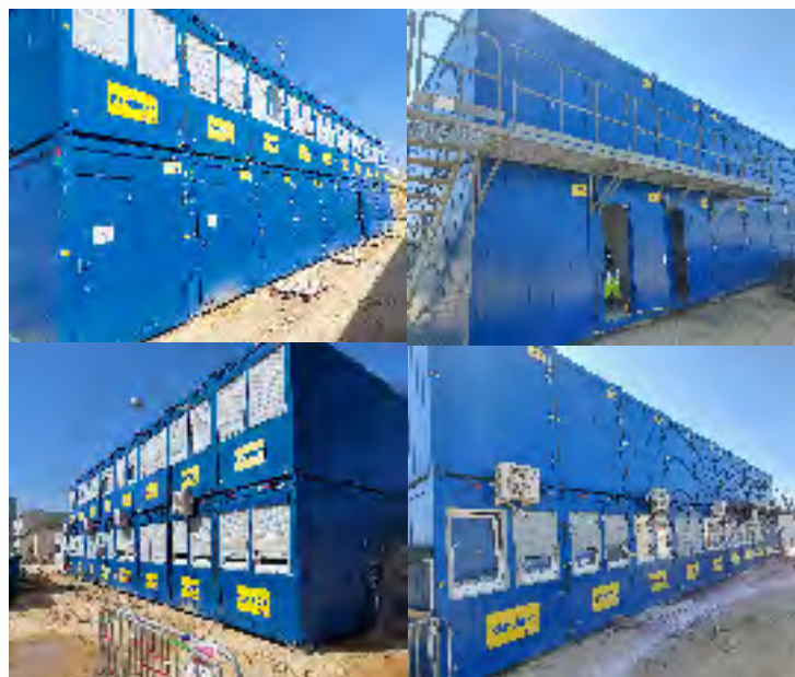
Fabryka akumulatorów SK hi-tech battery materials Poland
